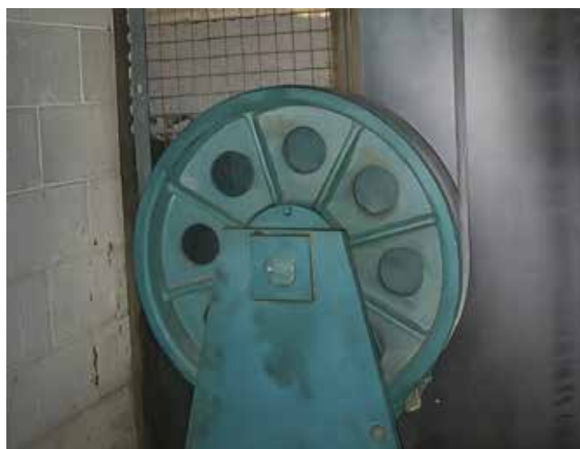
Fig. 15 AP bearings shown on typical elevator sheave application
